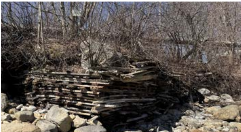
Photo #23 exposed demolition debris
