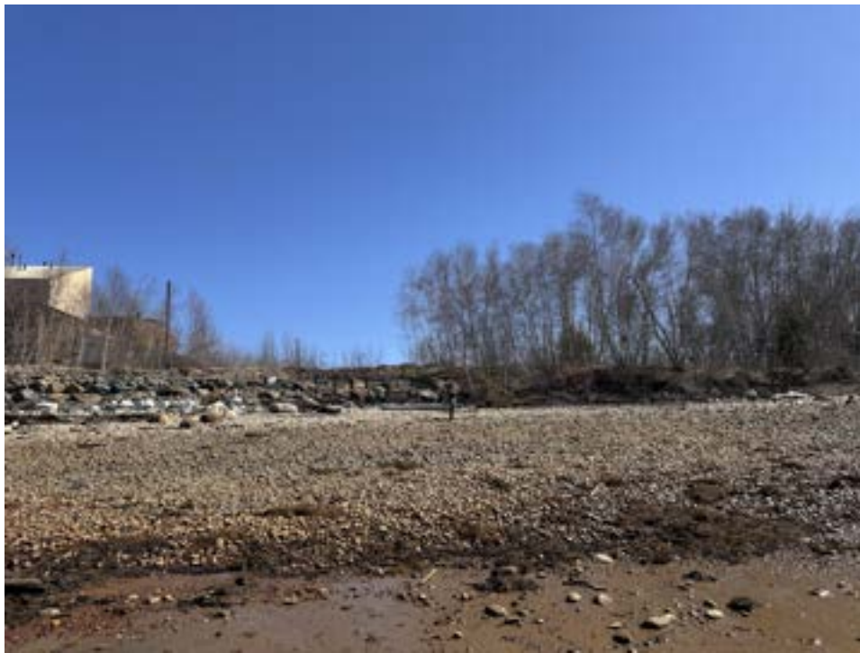
Photo #8 newly installed riprap, exposed plastic, grey powdery sediment 44.46454° N, 68.87976° W
