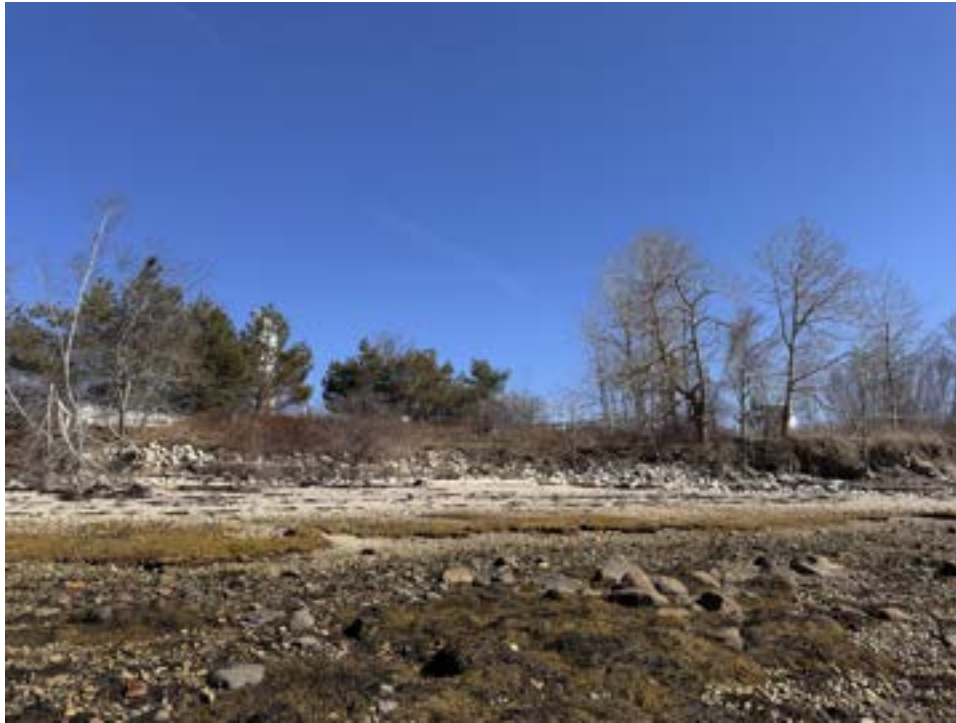
Photo #1. Overtopped riprap, highly unstable bluff. 44.46478° N, 68.88077° W.
