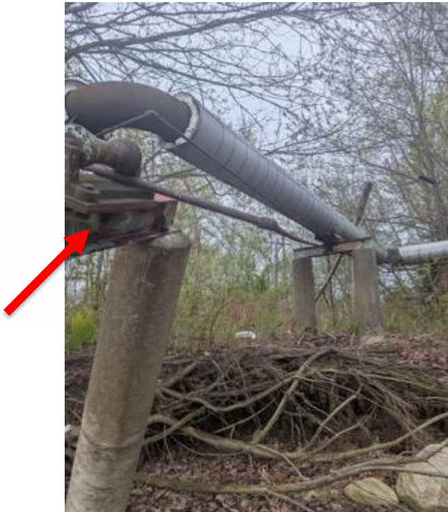
Field Sampling Photos 7 and 8: View of samples GAC-BM-C (red arrow), green paint on metal portions pipeline supports, and GAC-BM-D (blue arrow), black pipe wrap. Black pipe wrap is located along entirety of pipe and contains asbestos. The green paint is located throughout metal portions of pipeline supports and contains lead (5,700 mg/kg) and PCBs (3,300 ppm).
