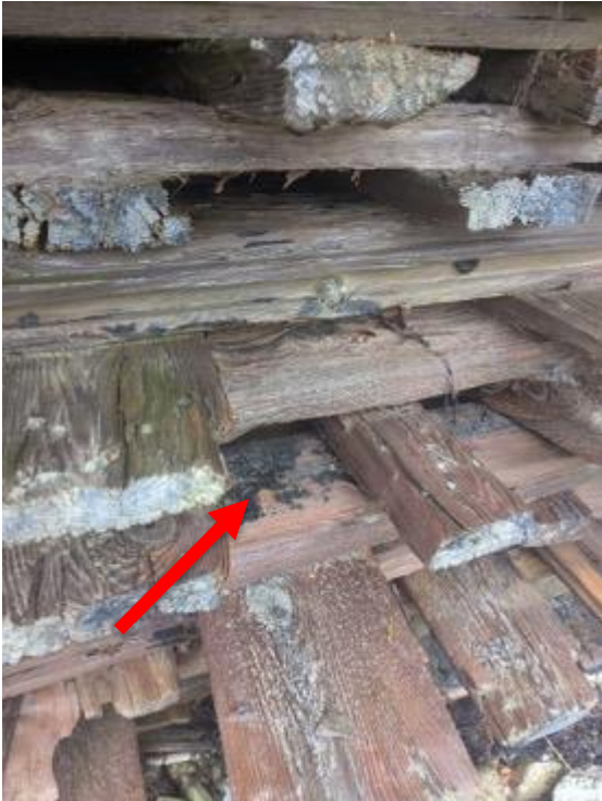
Field Sampling Photos 5 and 6: View of building material sample GAC-BM-B, black, tar-like coating on wood. This coating is located throughout this wood debris pile area.
