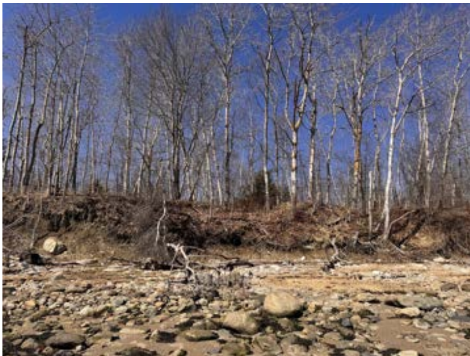
Photo #27 toe erosion on vegetated bluff
