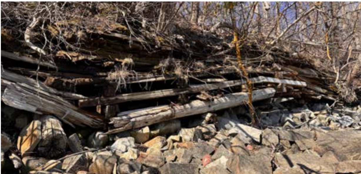
Photo #21 exposed demolition debris.
