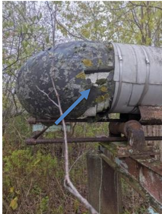
Field Sampling Photos 7 and 8: View of samples GAC-BM-C (red arrow), green paint on metal portions pipeline supports, and GAC-BM-D (blue arrow), black pipe wrap. Black pipe wrap is located along entirety of pipe and contains asbestos. The green paint is located throughout metal portions of pipeline supports and contains lead (5,700 mg/kg) and PCBs (3,300 ppm).
