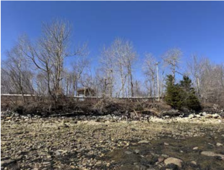
Photo #20 unstable bluff, inactive industrial pipe, exposed demolition debris under bluff 44.46547° N, 68.87788° W
